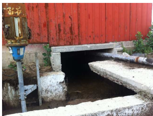
Figure 4. Canal concrete manure collection (farm picture)
