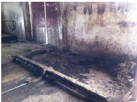
Figure 3. Plow scraper on the end of the barn (farm picture)
